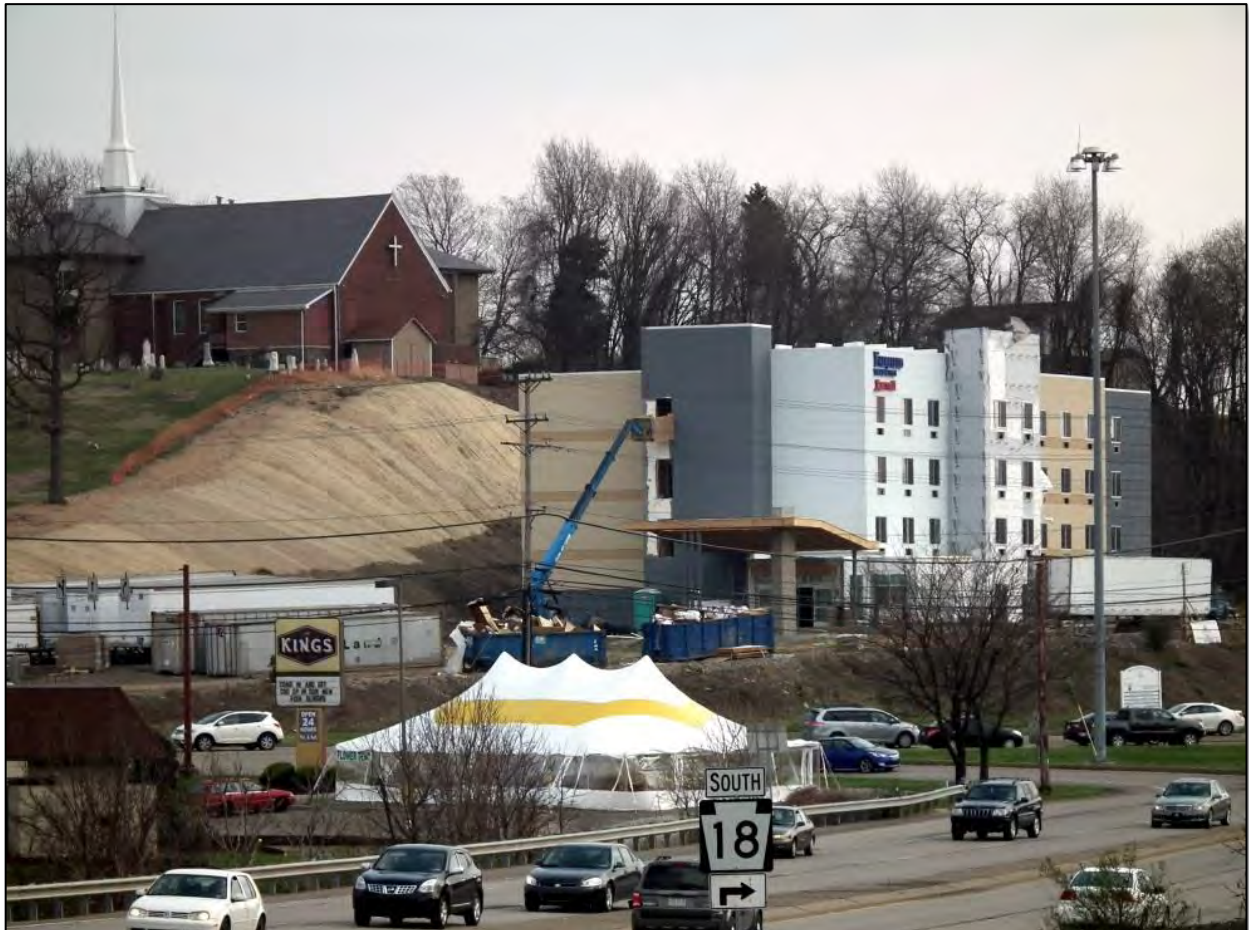
Figure 2.13: A new hotel is shoe-horned into a sliver of land between North Branch Presbyterian Church's cemetery and the intersection of PA 18 and Brodhead Road, Center Township - one mile from the proposed Shell ethane cracker plant. 4/28/14.
