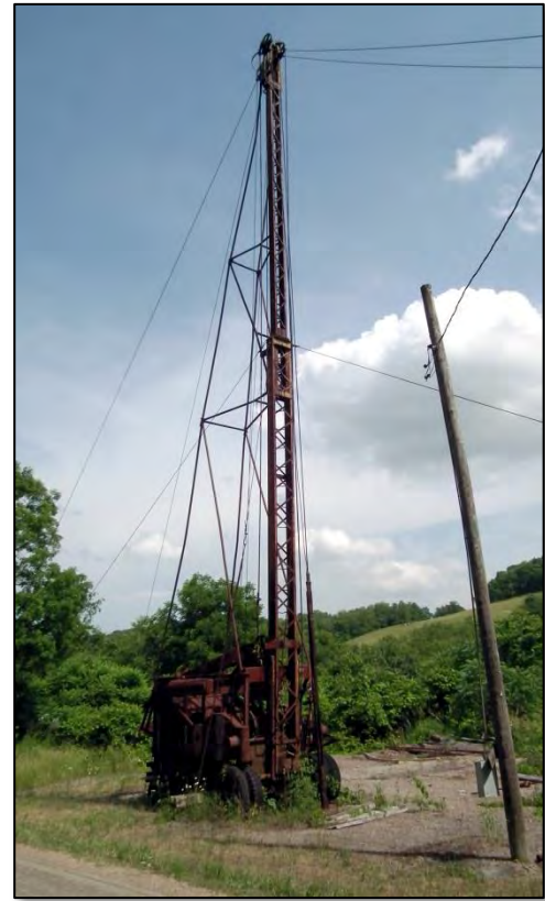
Figure 3.17: A Bucyrus-Erie cable tool drilling rig in Smith Township bears witness to the Region's industrial past. 6/18/2014.
