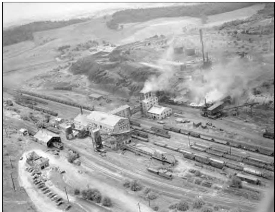
Figure 3.19: The Champion #1 coal washer in operation, June 27, 1946, serviced by the Montour Railroad. Photograph courtesy of the Archives Service Center, University of Pittsburgh.
