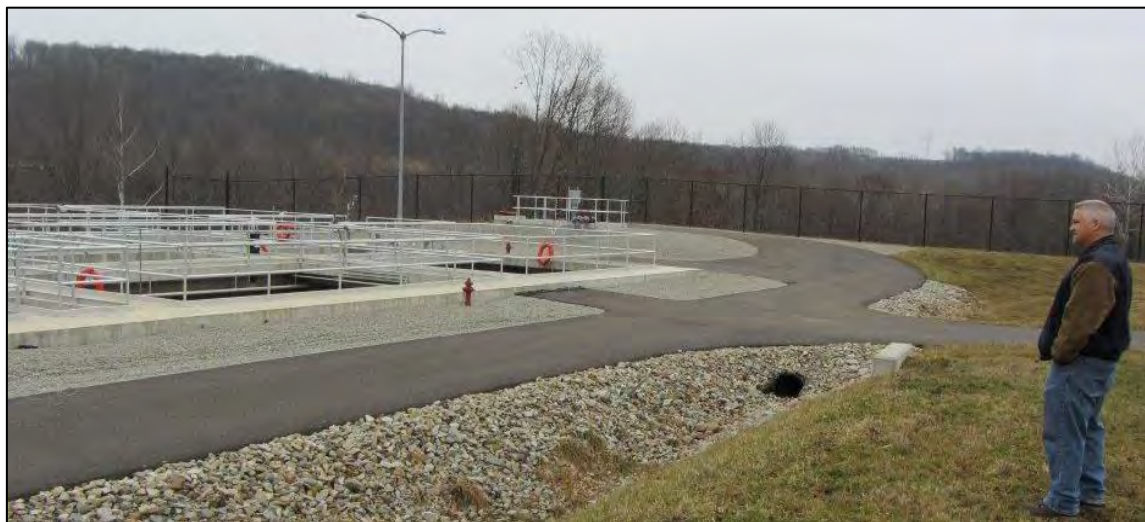
Figure 2.35: A gentleman admires the newly completed Independence-Cross Creek Township Joint Sewer Authority Treatment System plant expansion - January, 2012. Photo courtesy of Rachel Blosser, Manager, Cross Creek Township.
