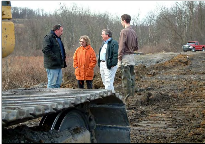
Figure 4.20: Former DEP Secretary David Hess (second from right) tours the JB1 Passive Treatment System under construction near Slak Lane in Smith Twp. L to R: Wayne Fuchs of Quality Aggregates, Margaret Dunn of Stream Restoration Inc., Hess, and Shaun Busler, also of SRI. Photo 12/12/2006.
