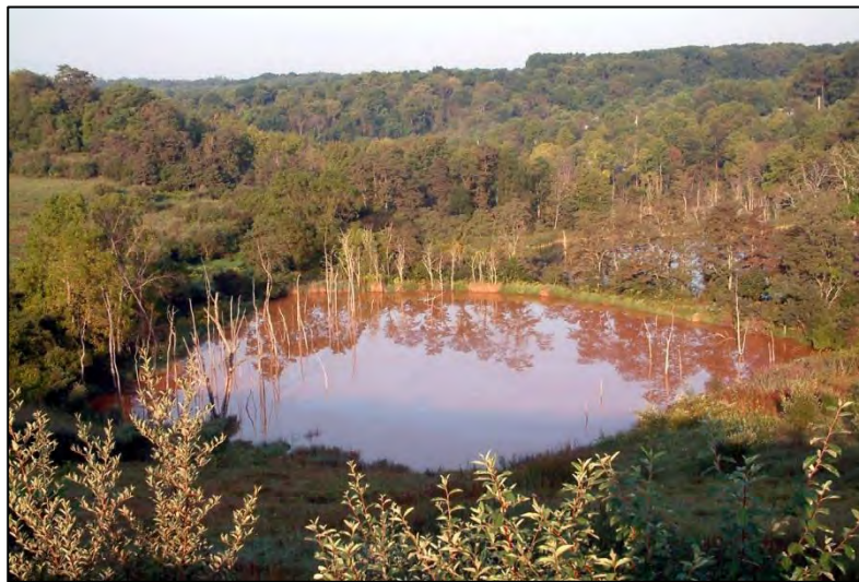
Figure 4.19: The upper two of a series of settling basins & wetlands that treat the Solar Mine Discharge, located near Bald Knob along I-576 in Findlay Twp. Initial treatment of this discharge takes place in a massive limestone-filled channel under the highway. Photo 6/7/2012.
