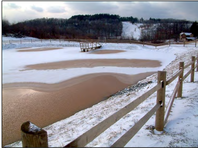
Figure 4.18: Upper settling basin of the Hamilton AMD Treatment System off Washington Rd. in Findlay Twp. The Burns-Hamilton Farmhouse is visible at far right. This National Register-eligible brick and cut stone home, built in 1841, was demolished in 2012. Photo 1/15/2004.
